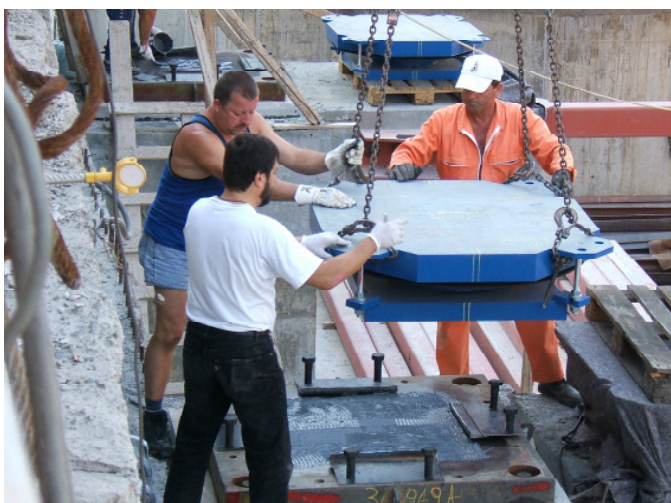
Fig. 3: SIP-installation on site
